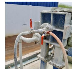
T joint at entrance of filter press with provision of valves for changeover between sludge pump and air from blower
