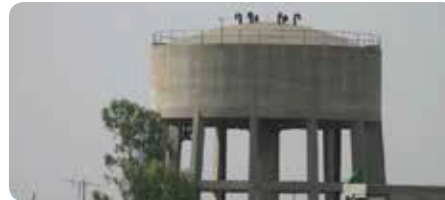
Domestic cement tanks, overhead cement tanks, and waterproofing of swimming pools.
