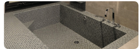
Waterproofing of sunken areas: Bathrooms, toilets, balconies etc.
